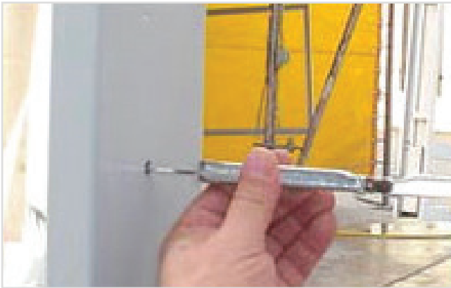
Adjust the pressure anchors.
