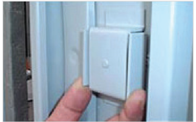
A properly adjusted pressure anchor is flush with the side of the frame.
